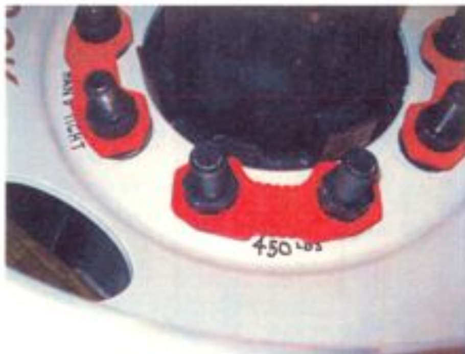
Figure 7 : Sample 10-03-C0152-5 installed on 450 ft-lb torque nuts
