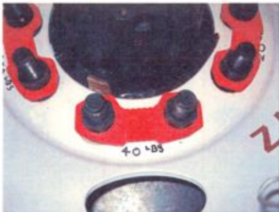
Figure 5 : Sample 10-03-C0152-3 installed on 40 ft-lb torque nuts
