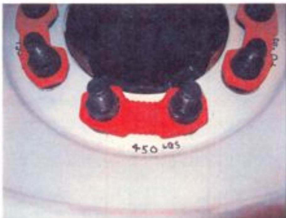
Figure 6 : Sample 10-03-C0152-4 installed on 450 ft-lb torque nuts
